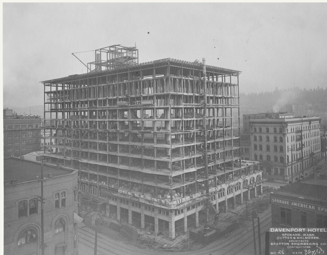
DAVENPORT HOTEL CONSTRUCTION 1913 JOEL E. FERRIS ARCHIVES L87-1.2.13
